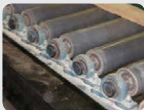
Overheating conveyor bearing
